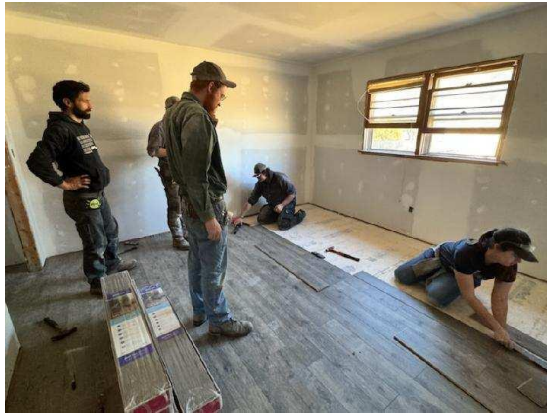
Above: The first weekend of February, I went to western North Carolina and helped work on a home that had been flooded during Hurricane Helene. We sanded sheetrock and installed flooring for the home. The crew after us will do texture, paint, and trim, then the home will be ready for the owners to move back.
